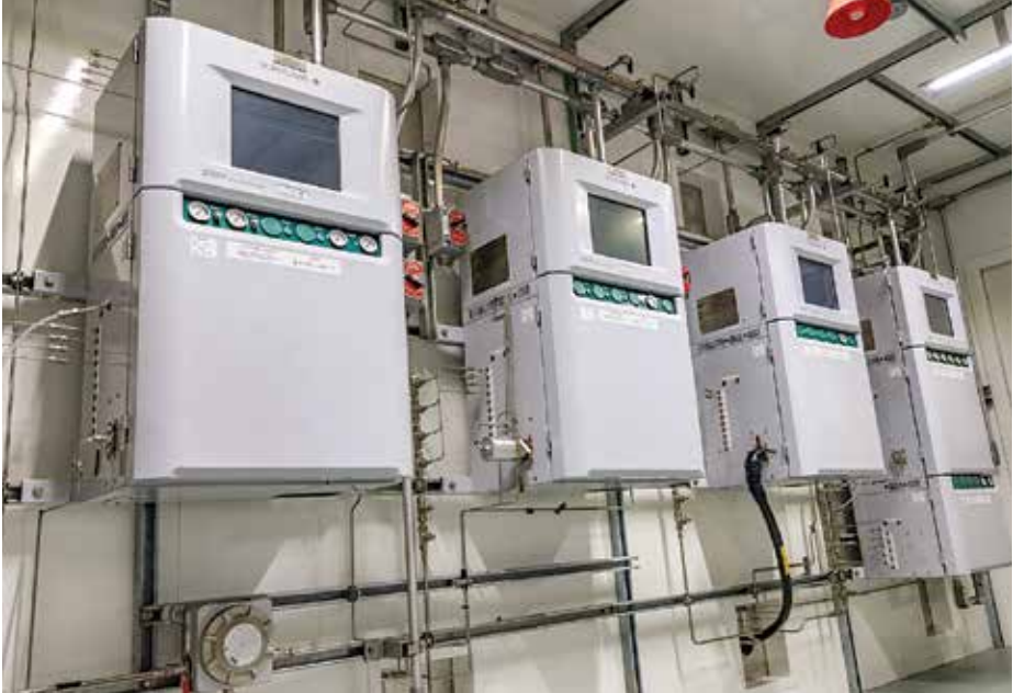
FIG. 1. A gas chromatograph, such as these Yokogawa GC-8000s, analyzes components in flare gas.
