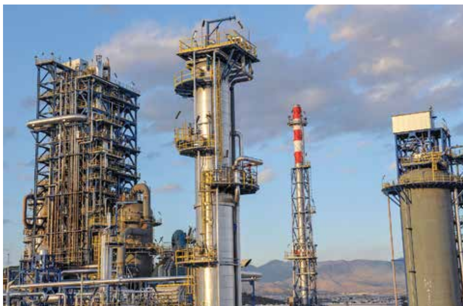
FIG. 2. ExxonMobil's FLEXICOKING™ technology unit at the Hellenic Petroleum Elefinsa refinery.
