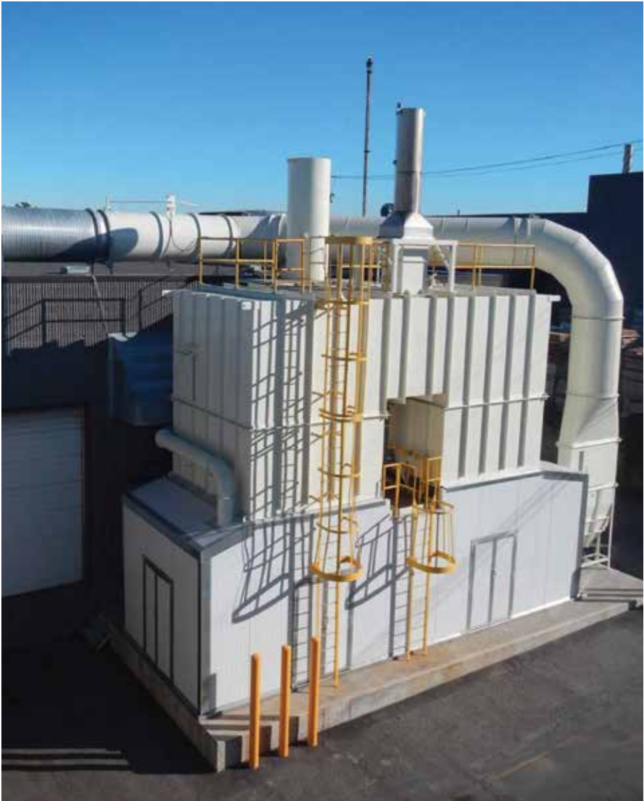
FIG. 2. Regenerative thermal oxidizers capture the heat from oxidation, which is retained by a ceramic media and is then used to heat and oxidize the process gas.
