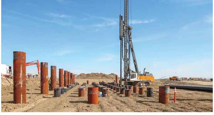
FIG. 1. Custom-designed helical piles have been used successfully on a number of recent petrochemical revamp projects.
