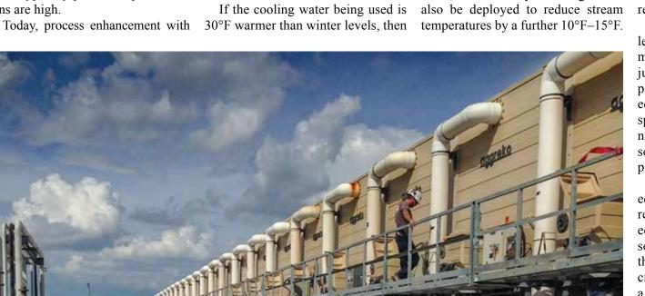
Closing the loop. A closed-circuit targeted cooling solution relies on a dedicated cooling tower or refrigerated chillers to drop process stream temperatures dramatically, even during the heat of summer. Installing rental heat exchangers, cooling towers or refrigerated mechanical chillers provides temporary, yet much-needed, relief from summertime heat (FIG. 1).
