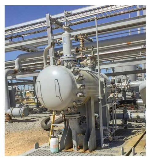
**FIG. 1.** With Pentair's HRT technology, the potential exists to dramatically improve hydrocarbon and solids separation from sour water without the need to expand existing residence tank capacity.
